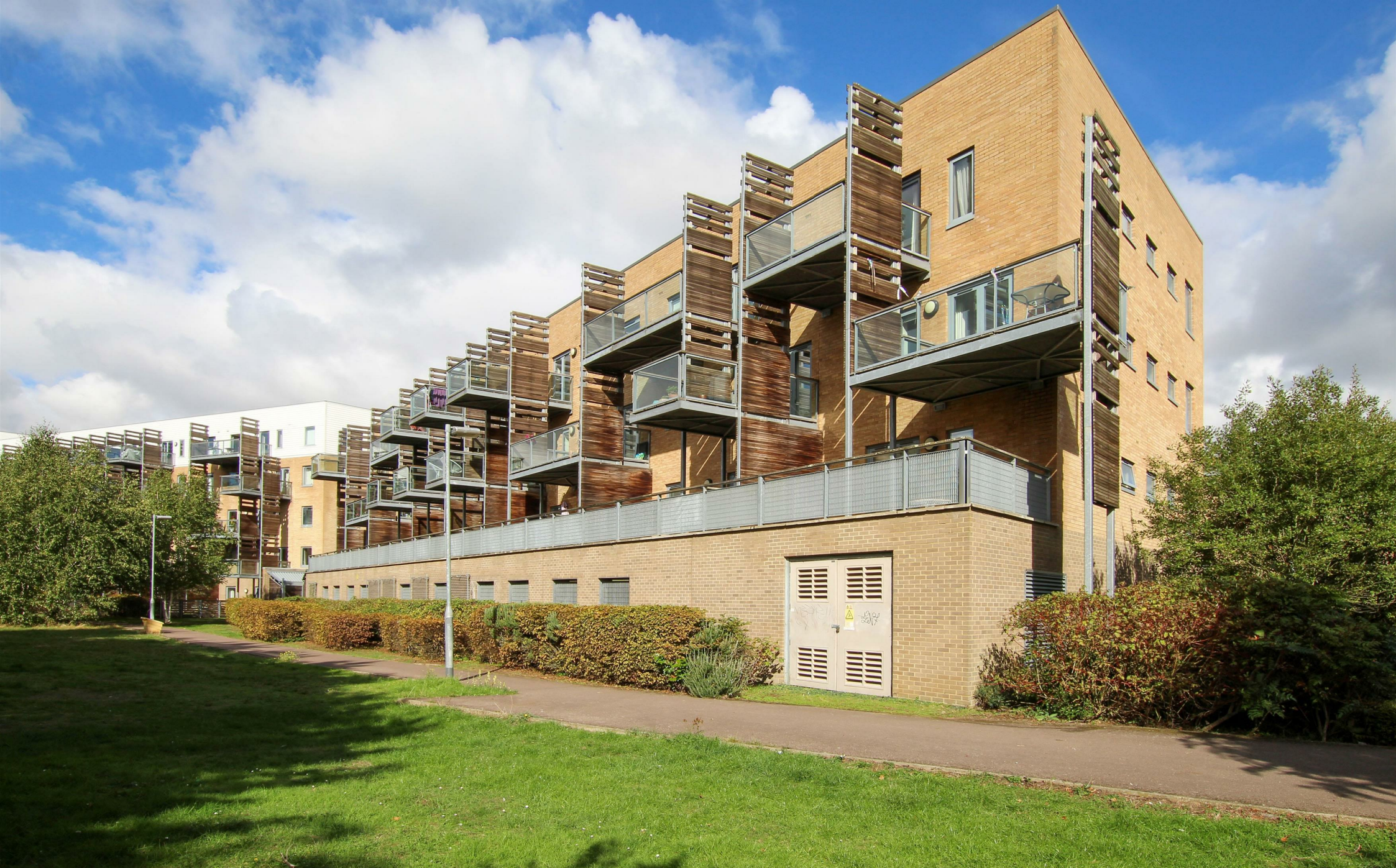
Bailey House, Rustat Avenue, Cambridge, CB1 3PG
